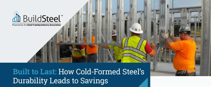
One of the major material advantages of CFS framing is that it is impervious to the environmental factors that typically threaten the integrity and lifespan of other framing materials. Because the material is resistant to corrosion, mold and vermin, it does not require costly treatments or repairs typical of other building materials.
