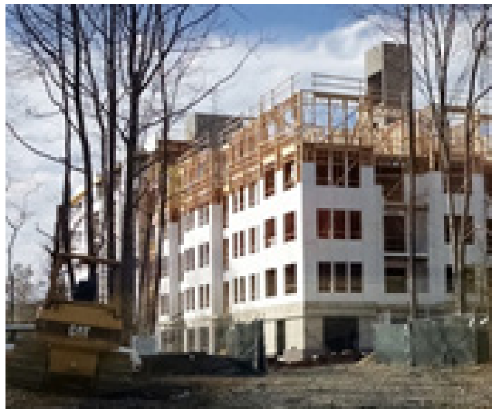
Wood framing over concrete "podium", Annapolis, MD
